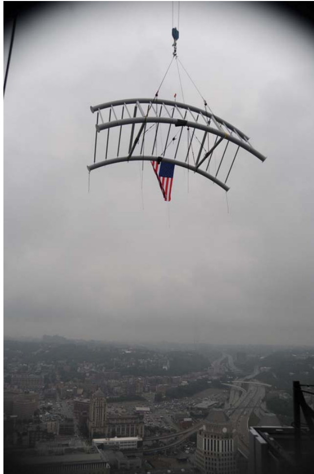
[PHOTO] An American flag hangs from the last piece of Great American Tower's tiara as it is lifted into place July 13. Great American Tower at Queen City Square is Cincinnati's tallest skyscraper at 665 feet.
